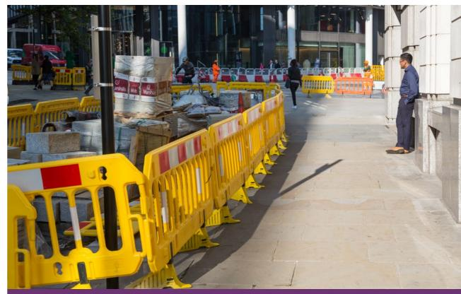
Good practice: tidy, correctly assembled and well-maintained barrier
