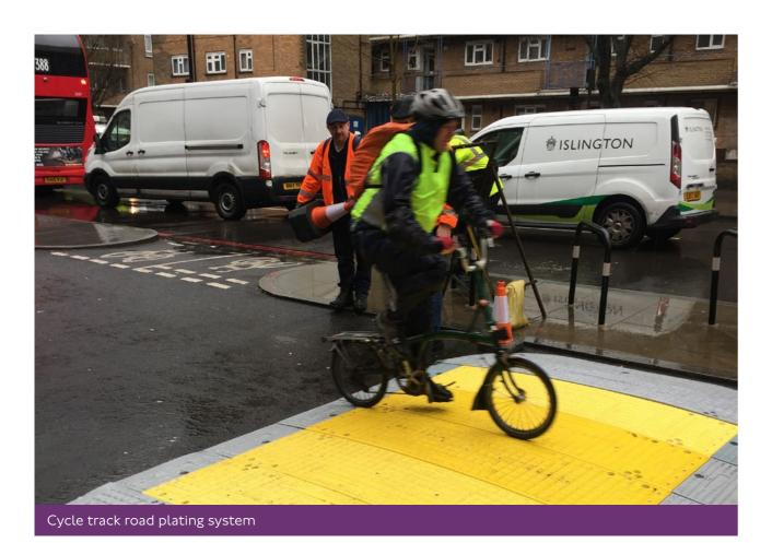
The London Cycling Design Standards advise that maximum linear ramp gradients should normally be between I:10 and I:20. It is recommended that the new surface of the hump is continued 500mm beyond the ramp into the existing carriageway surface to produce a smoother profile.
